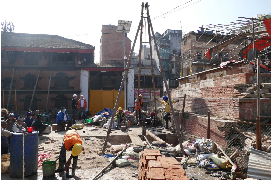
Figure 8. Borehole drilling being undertaken adjacent to the Trailokiya Mohan Temple, Hanuman Dhoka Durbar Square. (Image: Durham UNESCO Chair)
