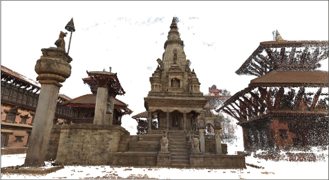
Figure 12. Web-scraped image for the Vatsala Temple in Bhaktapur's Durbar Square, Kathmandu, Nepal which collapsed during the 2015 Gorkha Earthquake. (Image: Bradford University)
