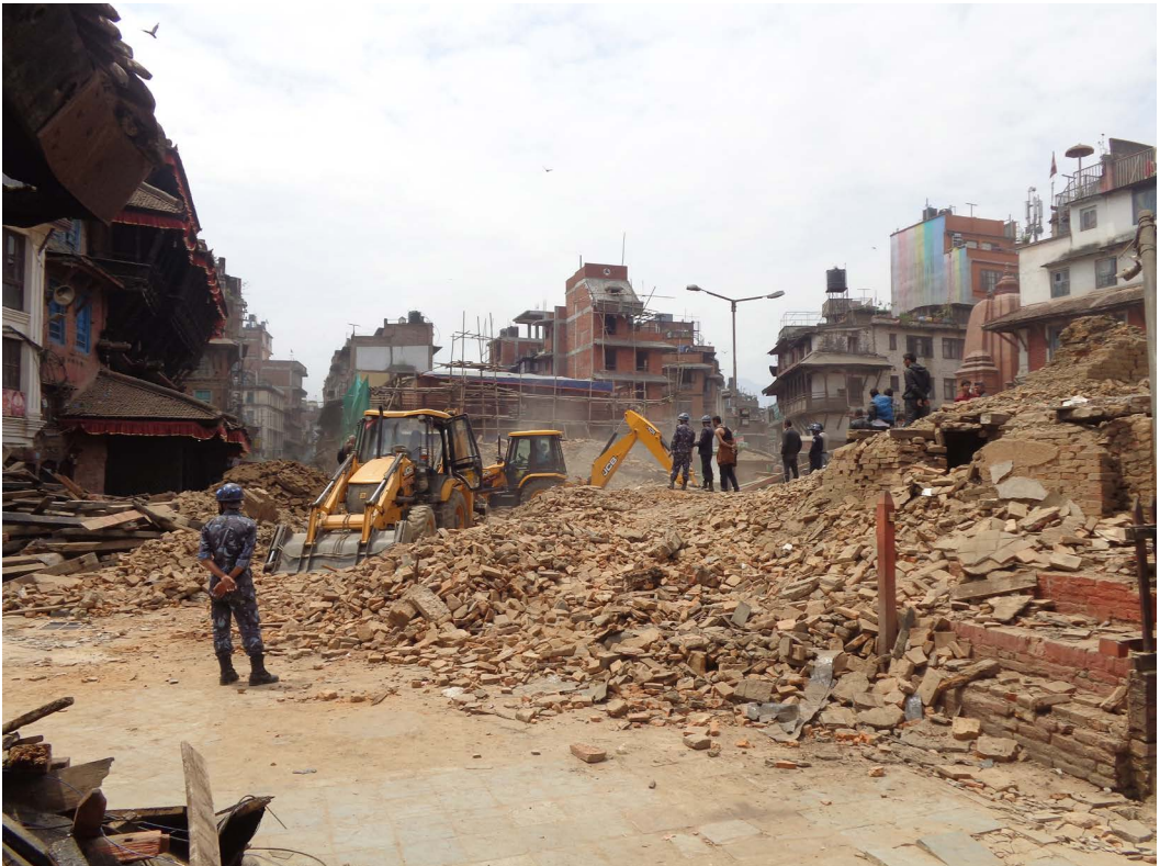
Figure 3. JCBs clearing debris at the Kasthamandap on 26 April 2015. (Image: Kai Weise)
