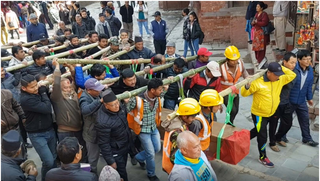
Figure 1. One of the newly carved central timber columns of the Kasthamandap being transported by the community to the monument site. (Image: Kai Weise)
